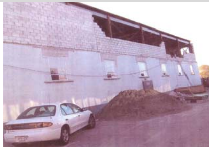
CONSTRUCTION OF THE SECOND FLOOR
